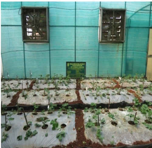
Inside view of fan and pad system
