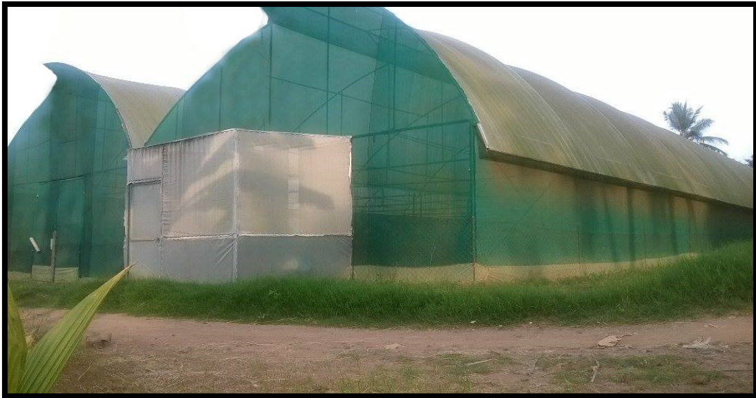
1A. Naturally ventilated saw tooth type polyhouse located in Instructional Farm, Vellayani
