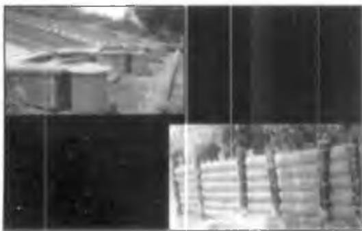
Use of coir geo-textiles for varying slopes and river bank protection
