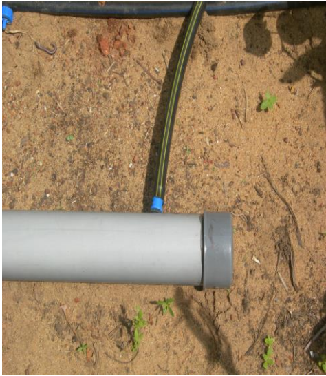
A) Lateral connected to main
