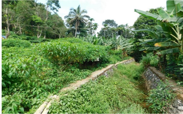
Stream Bank Stabilization
