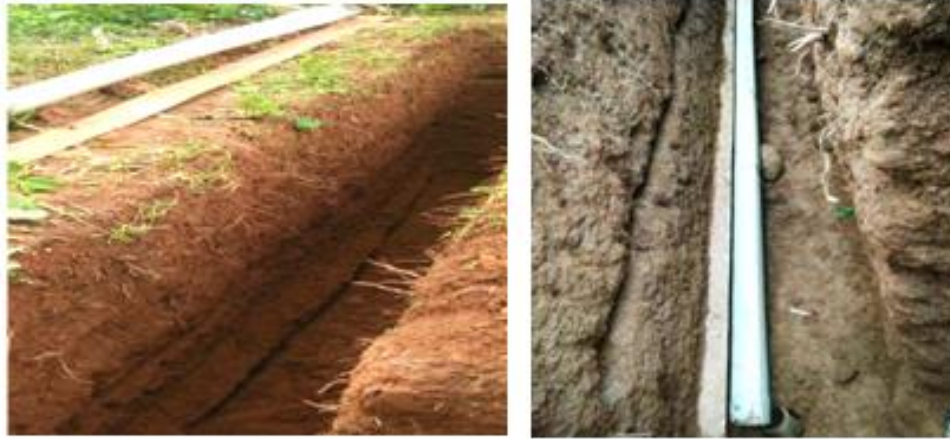
Plate 3.1 Installation of experimental set up in site 1
