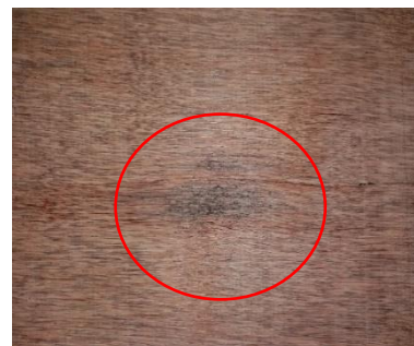
Plate 20: Example of veneer decay
