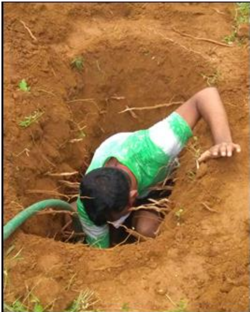
Fig. 3.18. Installation of CS650 Soil Moisture Sensor
