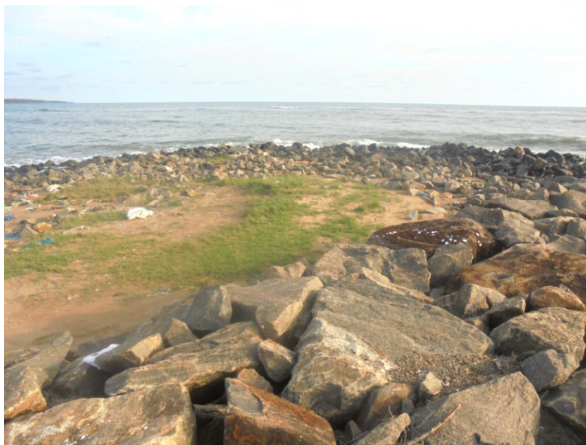
Plate 4.2 Parts of old and renovated breakwater at Bharathapuzha river mouth
