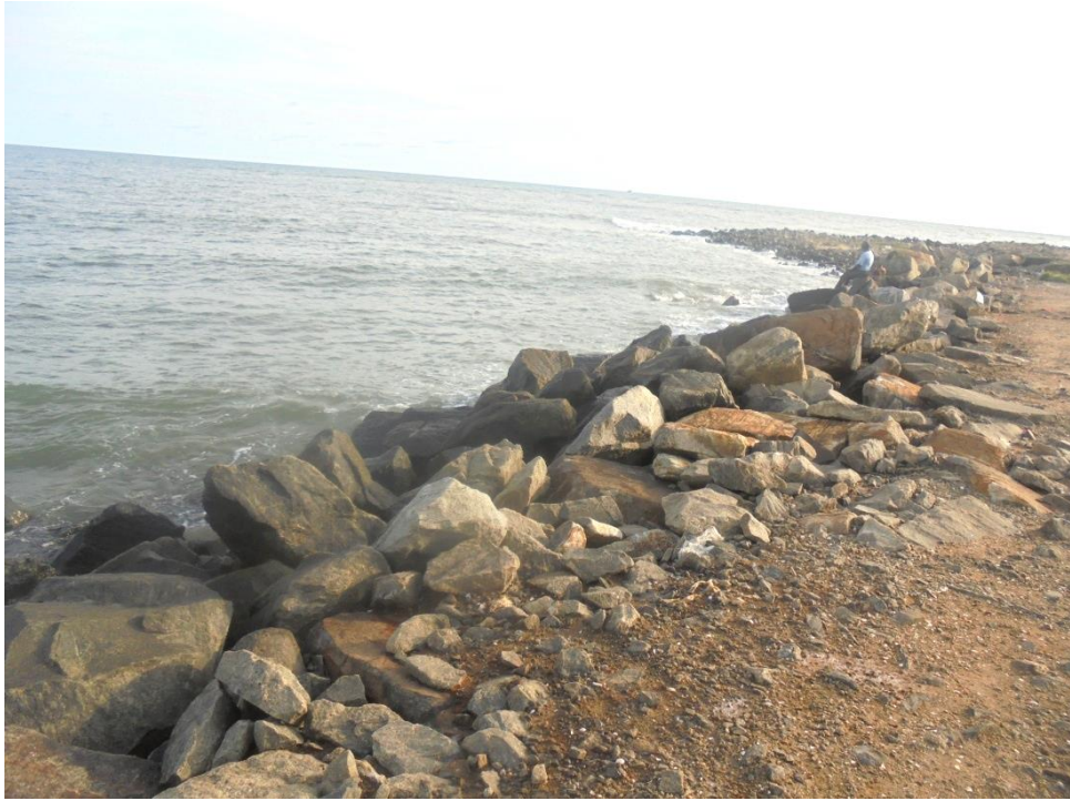
Plate 4.3 Breakwater at Bharathapuzha River mouth
