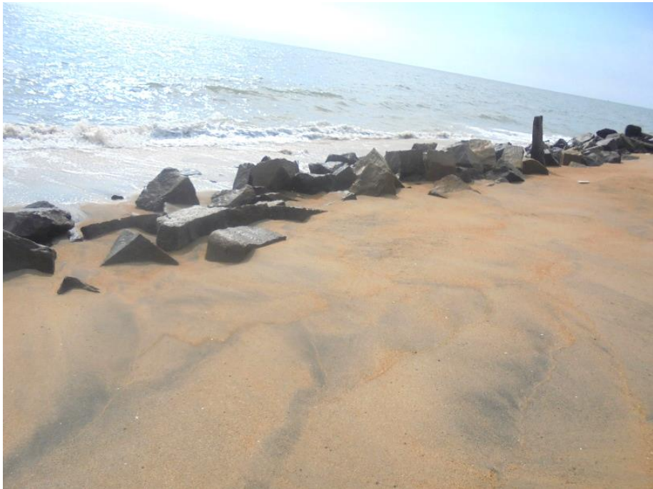
Plate 4.8 Remaining part of old structure along Palappetty coast
