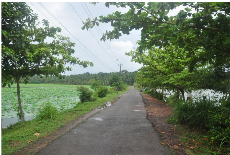
Plate 35. Vavvamoola Bund Road
