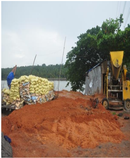
Plate 28. WSS to Kovalam (Under construction)
