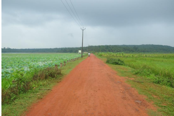
Plate 33. Reservoir Bund Road
