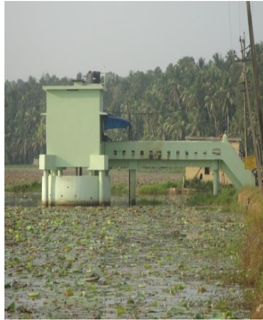
Plate 29. CPWD pumping station
