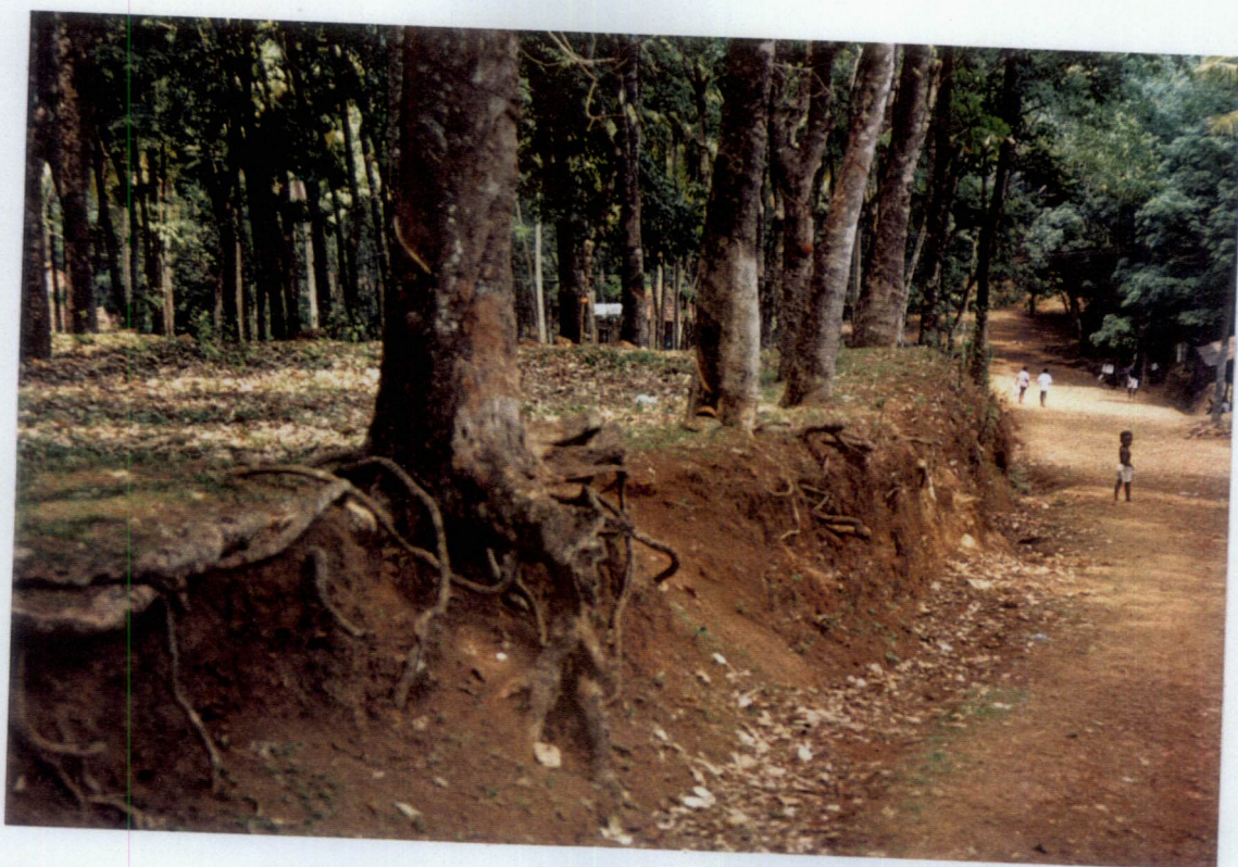
Plate 9 . Exposure of roots due to soil erosion on a hillslope (Pampadi Panchayat)
