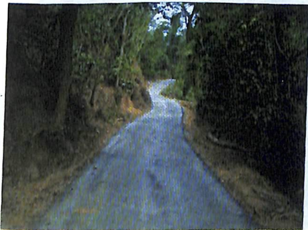
KATTEKKAD - PULIYARA ROAD
