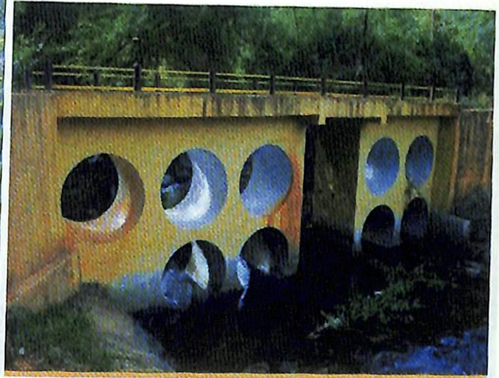
PIPE BRIDGE IN KARUVARA
