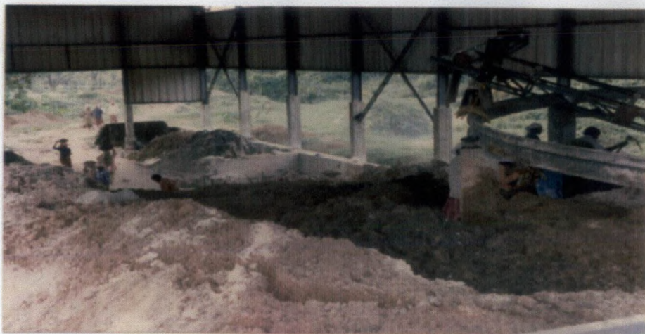
Accumulation of filtered sludge- 7 to 10 t/day
