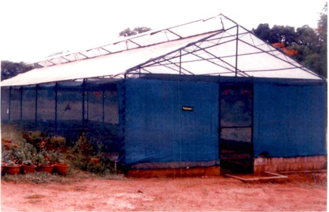
Plate 6. General view of the structure
