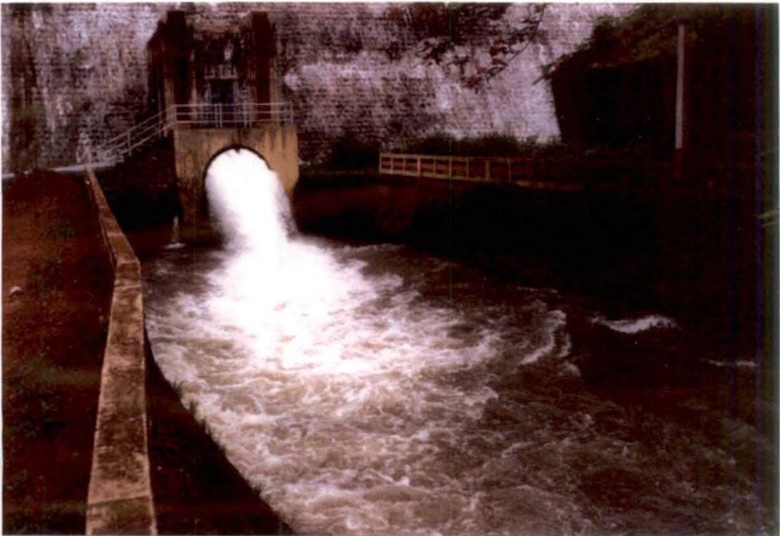
Plate 3.2 Right Bank Canal- A view from the dam
