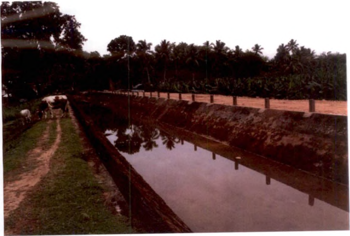
Plate 4.5 Lined canal in head reach
