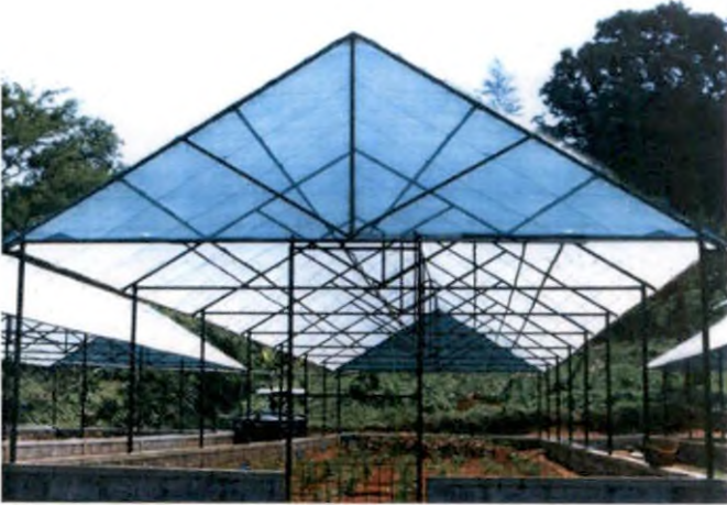
Plate 1. Naturally ventilated polyhouse
