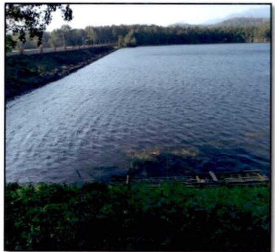
C) Peruvaripallam dam
