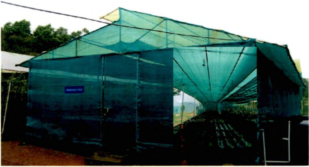
a) Top ventilated rain shelter
