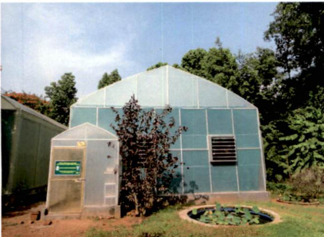
Plate 2a. General view of fan and pad system (FP)
