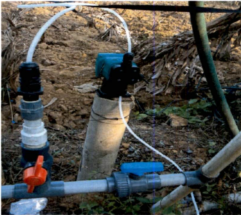
Plate 3. Fertilizer injector used for fertigation
