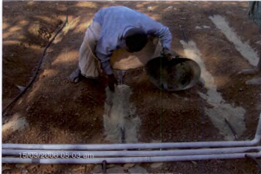
Plate 3.10. Porous Pipes with Sand Envelope
