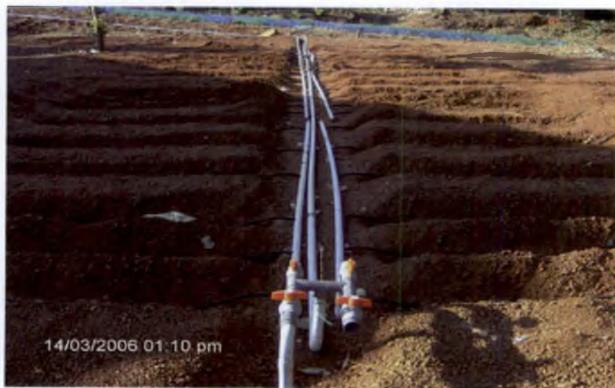
Plate.3.9. .Porous Pipes Installation
