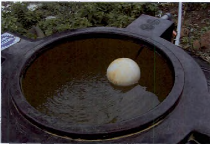
Plate 3.7. Feeder Tank with Float Valve
