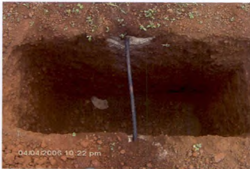
Plate 3.12. Moisture Distribution of Porous Pipes
