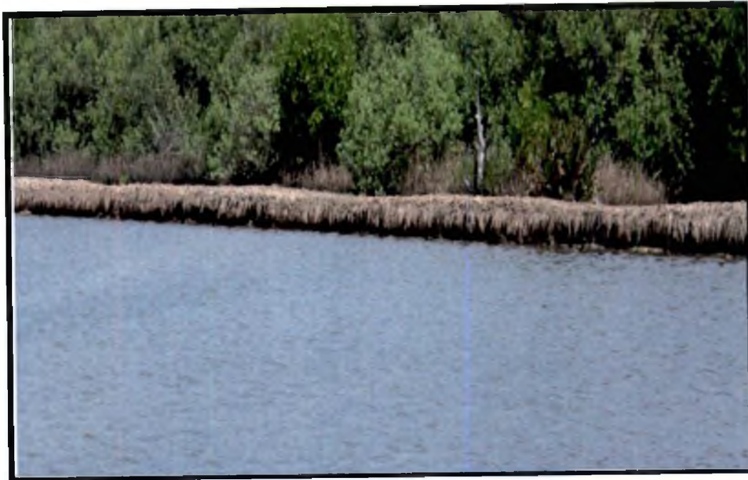
(a) Bunds constructed for prawn filtration
