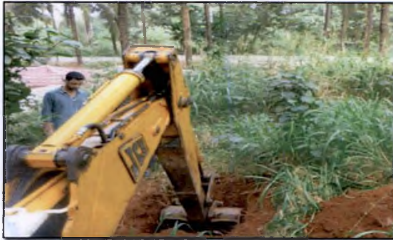
Plate 7. Digging pit for soil carbon sequestration assessment
