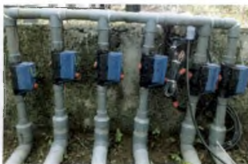
Plate 3.13 Series of solenoid valves
