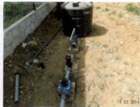
Plate 3.12 Control head components
