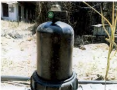
Plate 3.11 Disc filter
