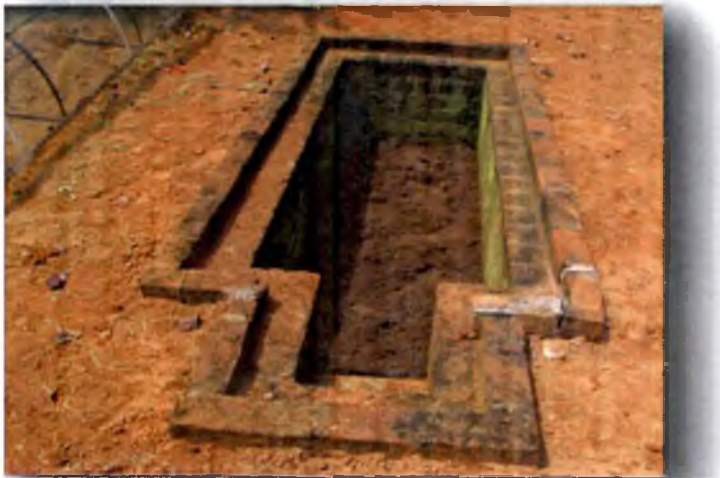
Plate 5. Trench with coirpith spread on the floor
