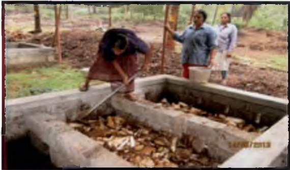
Transfer of residues to tanks
