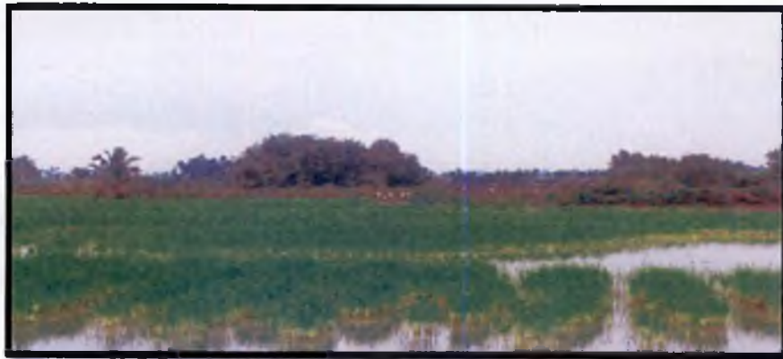
Plate 2: Mound dismantling stage
