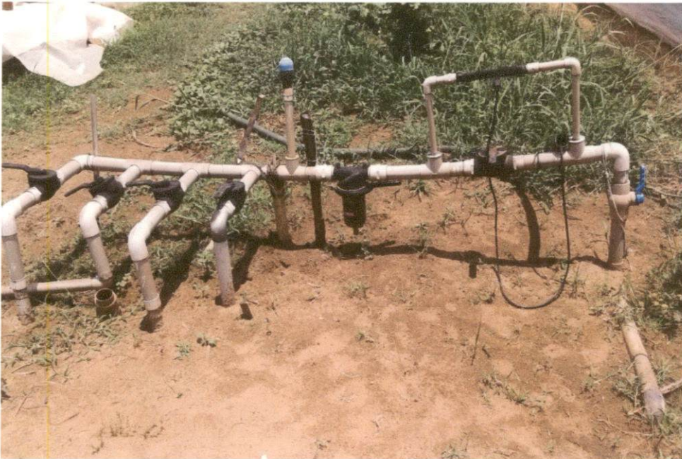
Plate 3.6 Control system of drip irrigation
