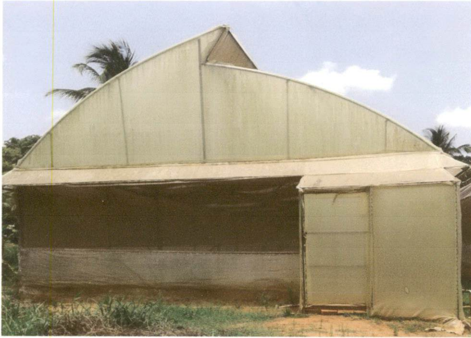
Plate 3.1 Naturally ventilated polyhouse
