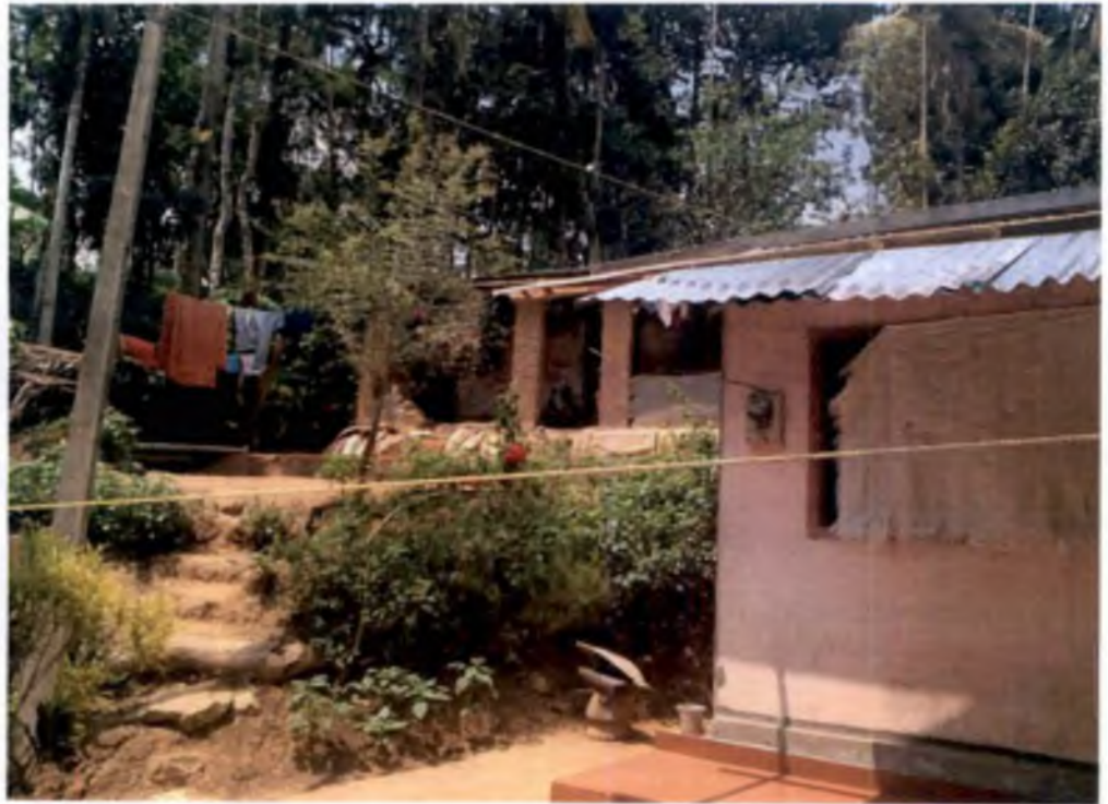
Plate 4. Tribal houses in Thirunelli panchayath
