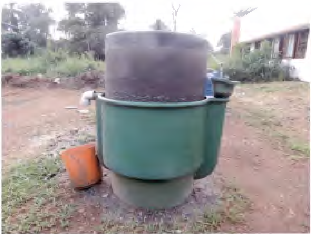
Figure 10. Floating gas holder type PBP with water seal
