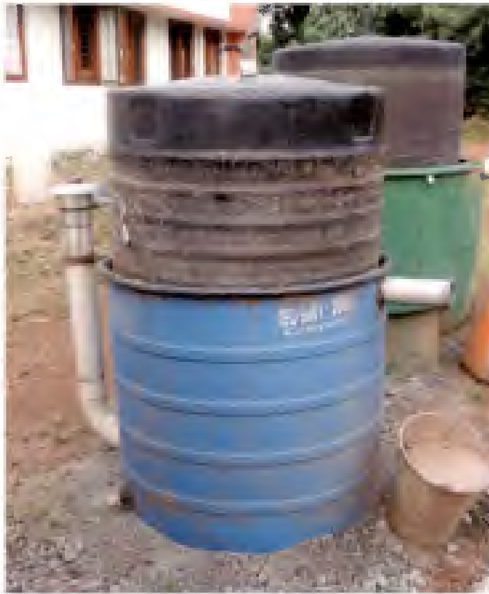
Figure 8. Floating gas holder type PBP without water seal
