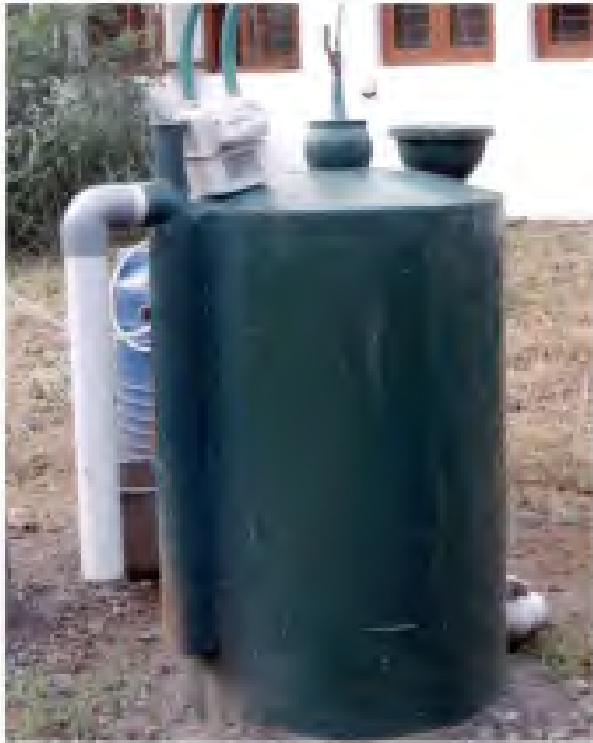
Figure 12. Fixed gasholder type PBP
