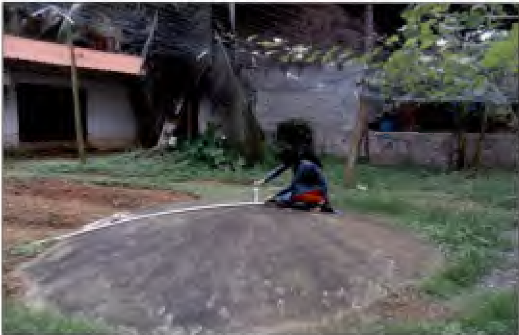
Figure 8. Biogas plant in the dairy farm
