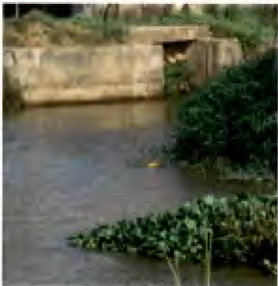
Site 3. Reservoir bund
