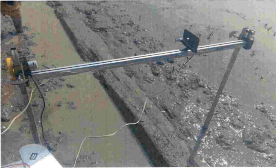
Plate 3.14 In situ measurement of the bund profile
