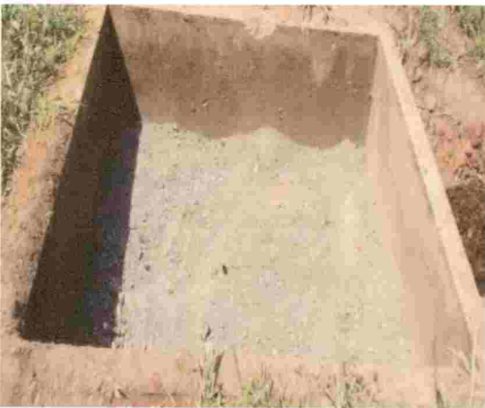
Plate 3.6 Drainage media filling
