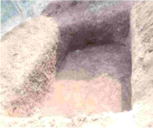
Plate 3.4 Pit for lysimeter installation
