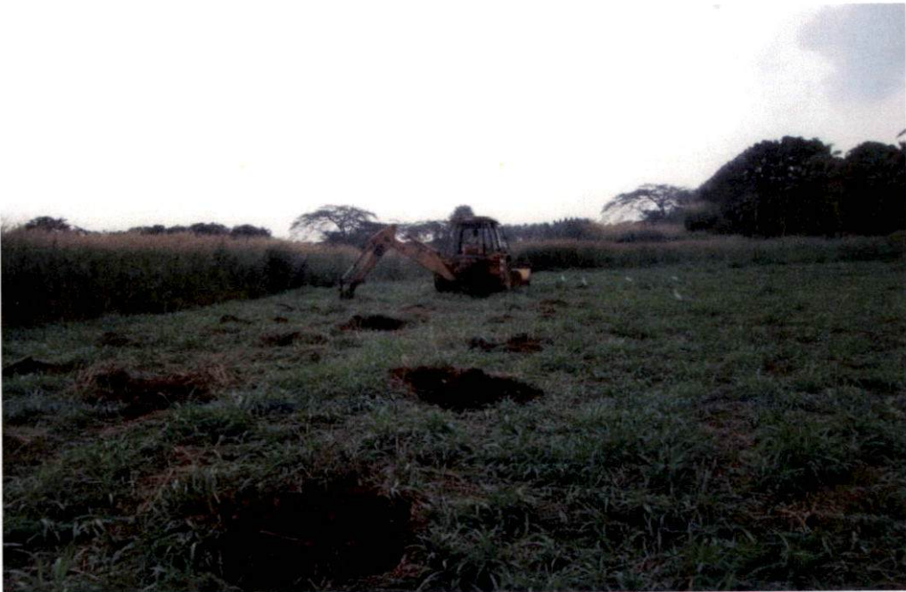
Plate13. Preparation of planting pits
