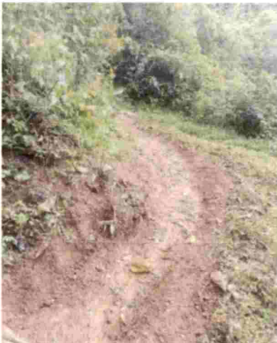
Plate 3.1:Earthwork in Boundary
