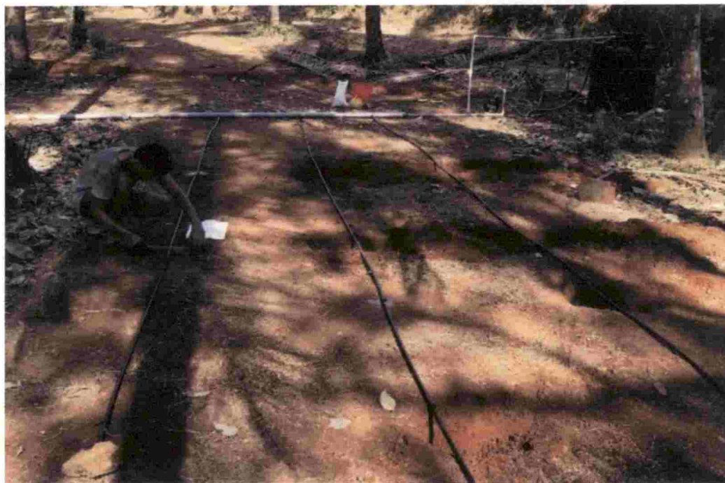
Plate 3.15 Setup for Continuous Drip Irrigation System
