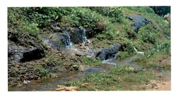
Figure 26. Leakage from main canal
