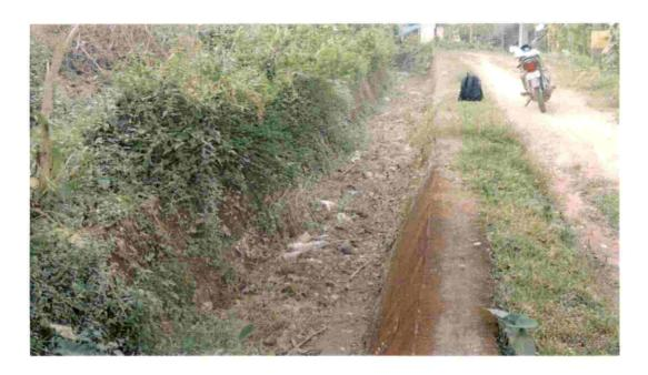
Figure 28. Improper maintenance of branch canals
