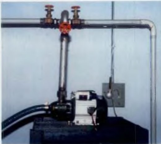
Test setup- Pump, pipe and control valves
