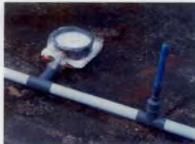
Floppy sprinklers - JFPP connected directly to the main line and JFLP on riser tube
