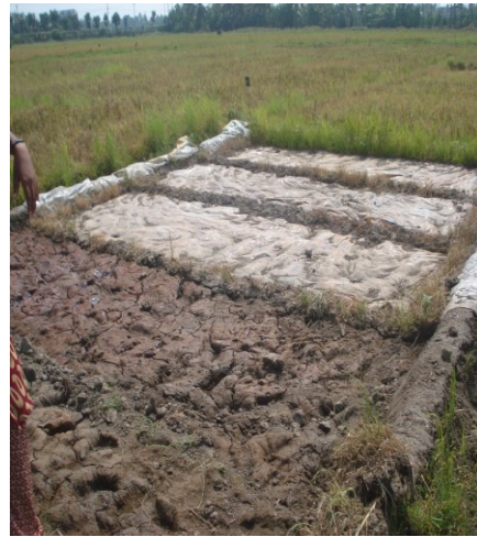
C. Stage wise removal of sheet
