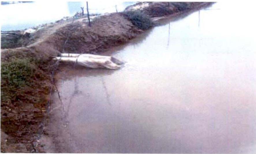
Plate 6 L.vannamei pond without proper inlet and crab fencing
