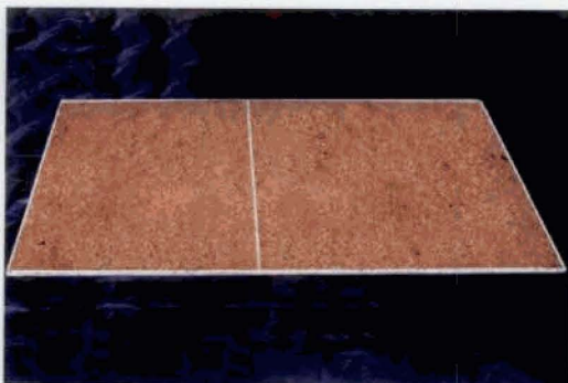
Covering with thin film of rooting media
