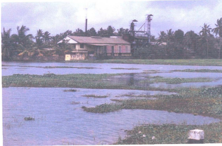
Plate 7. Conversion of paddy field for industrial purpose
