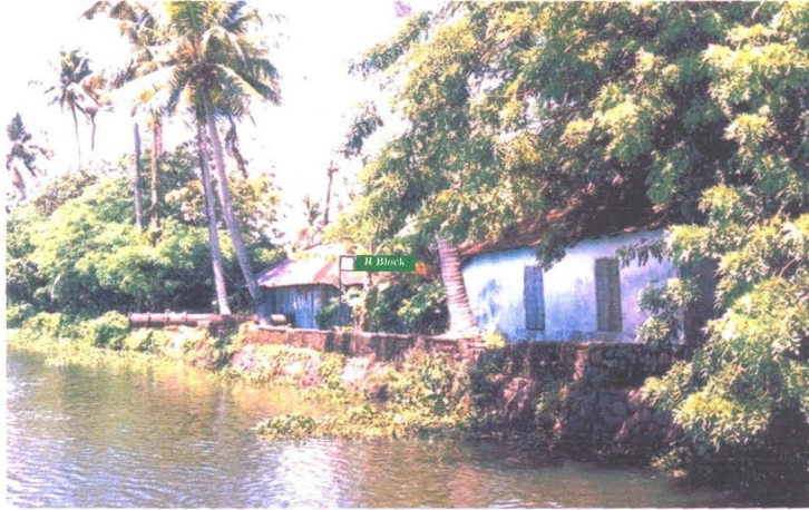
Plate 13. View of 'R' block showing the permanent non-submersible bund and centrifugal pump to bail out water*
