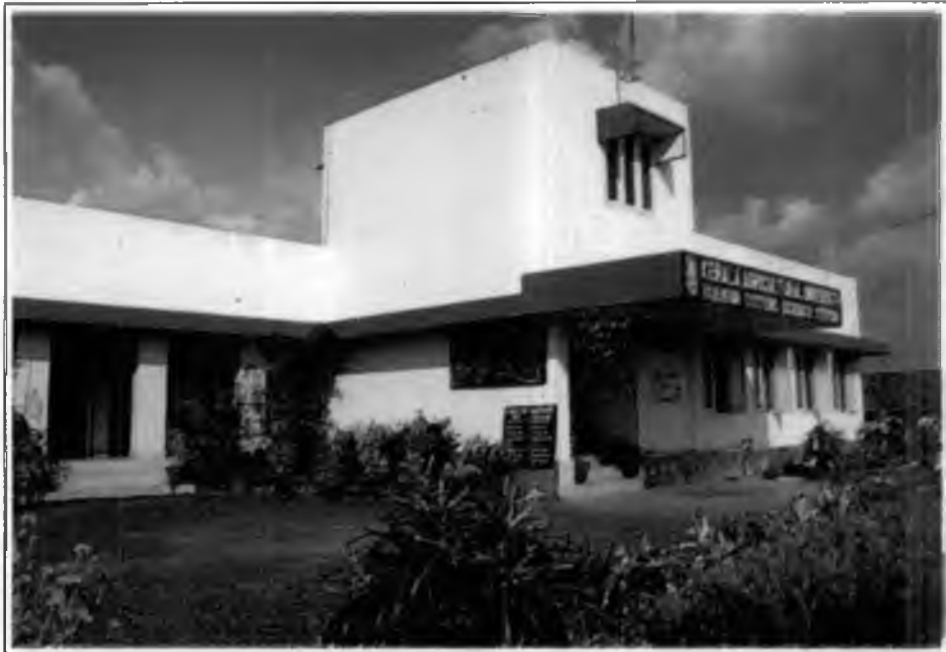
Field Laboratory cum Office building, Farming Systems Research Station, Kottarakkara.
