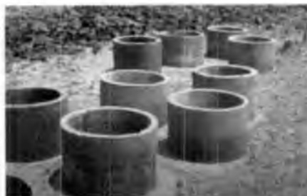
Figure 4.13 Pre-fabricated concrete rings for collection sumps
