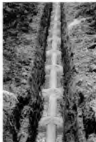
Figure 4.20 River sand as filter material
