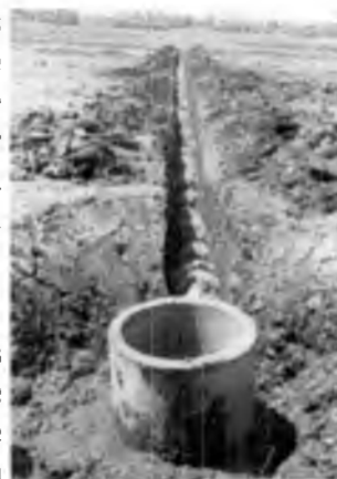
Figure 4.12 Laid out drain in the field
