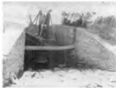
Figure 3.16 Typical field installation of Petty and Para (locally made axial-flow pump)
