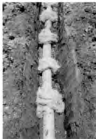
Figure 4.19 Coir fibre as filter material
