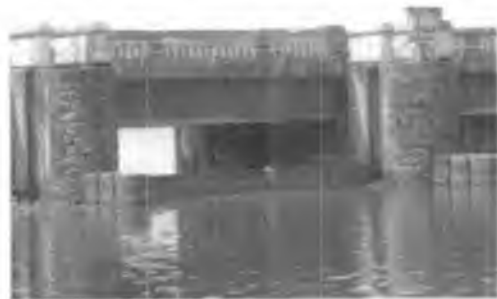
Figure 3.11 Thottappally spillway with its shutters closed
