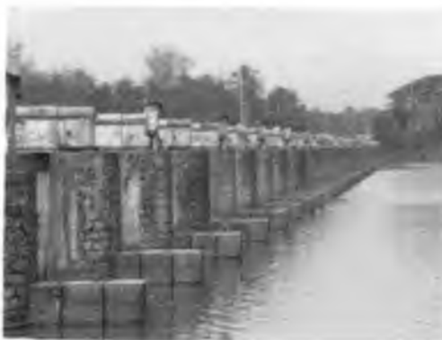
Figure 3.10 Thottappally Spillway, an important flood relief structure
