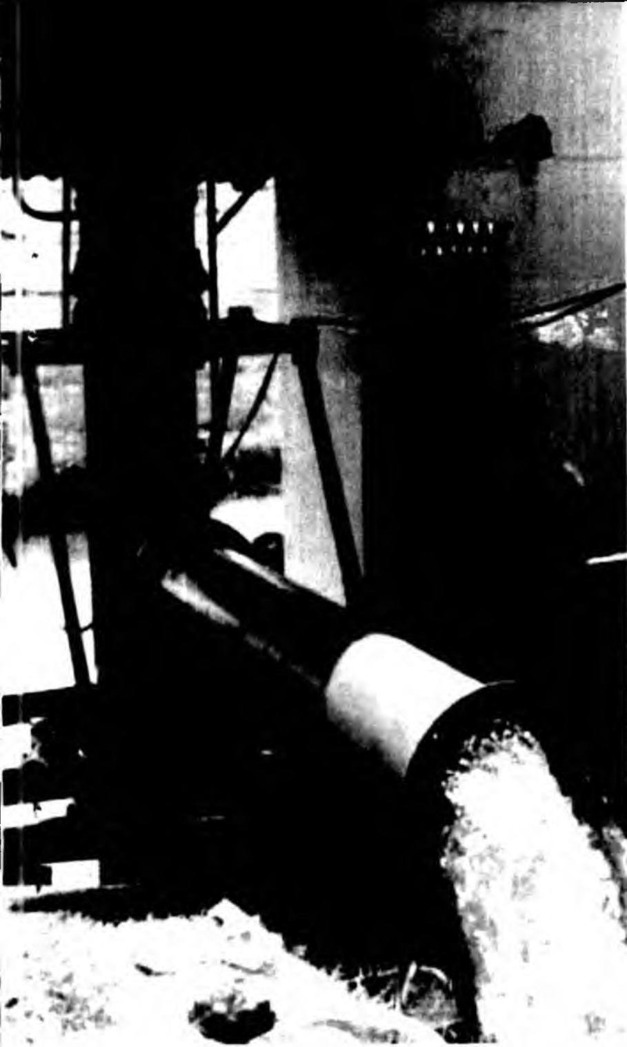
Vertical axial flow pump installed at Kole lands of Karalam, Thrissur
