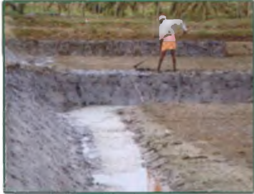
Strengthening outer bunds
