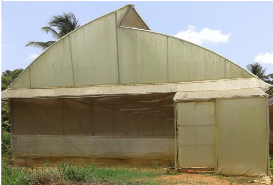
Plate 3.3 Naturally ventilated greenhouse
