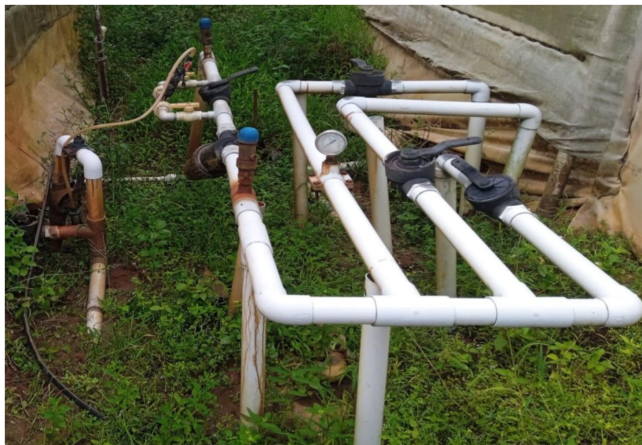
Plate 3.7 Control system of drip irrigation
