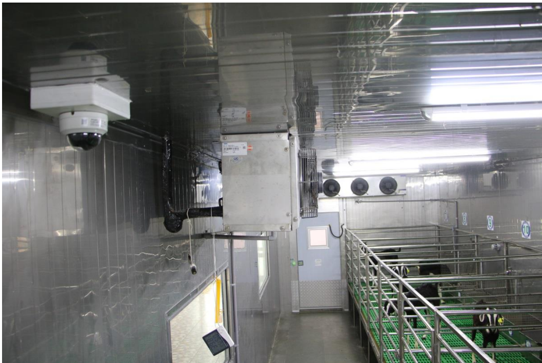
Plate 3.3: Inside view of Climate chamber; Sensors for recording weather parameters like temperature and humidity.
