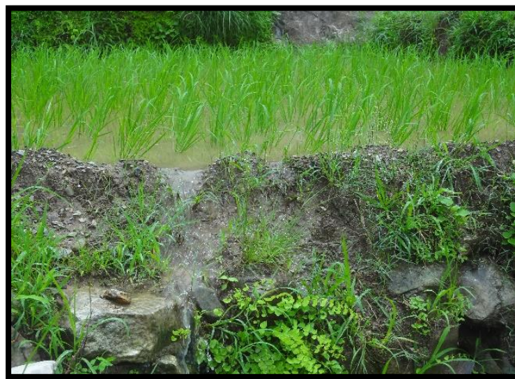
Figure 46. Breaking of terraces during monsoon
