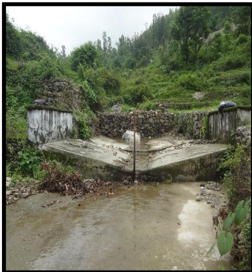
Figure 8. Weir structure at the outlet Figure 9. Digital Water Level Recorder
